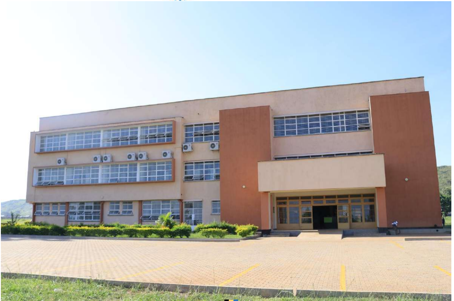
Engineering Library @ Busitema – Front View
